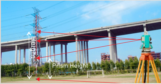
Remote Elevation Measurement
